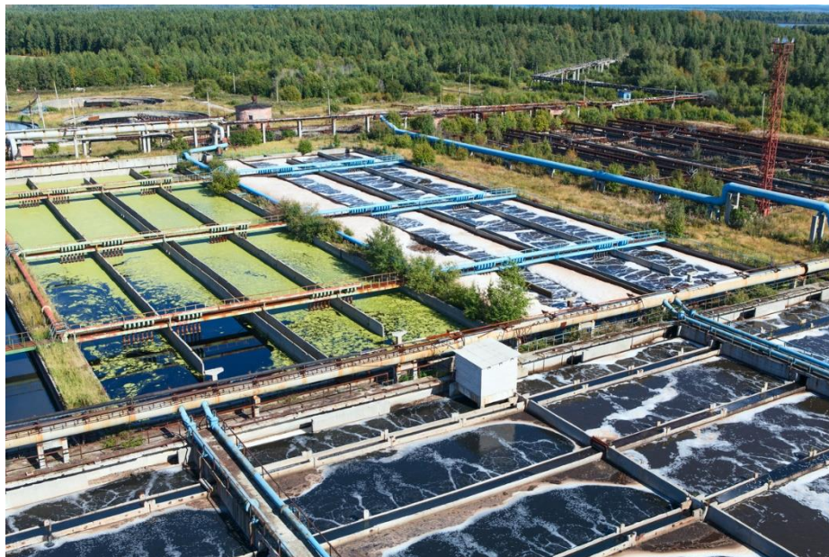
Figure 5.1 - Open pond biological treatment [65]
